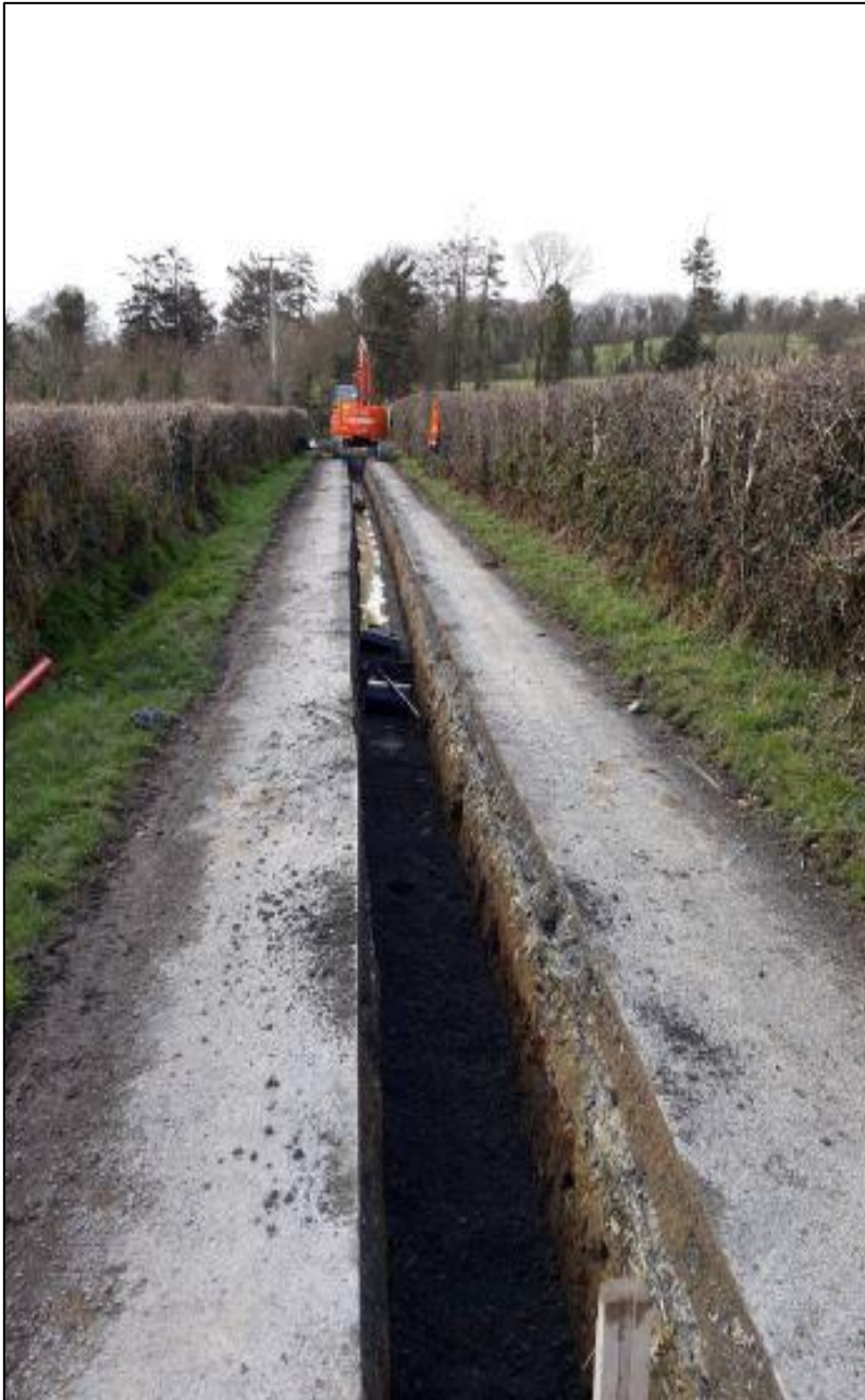
Plate 2.3: Typical Trench Construction within roads
