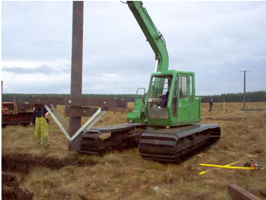
Plate 2.2: Photograph of a Typical 20 kV Pole with Excavation
